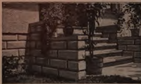
Confronted with a Shortage of Cement Blocks, the Builder Nailed V-Shaped Wooden Strips to the Forms with the Pleasing Result Shown Here
